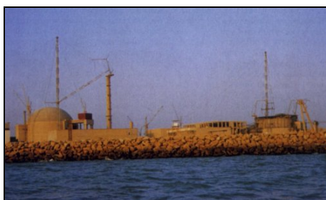
Figure 4 Construction of the Bushehr reactor.
