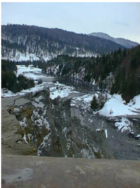
Figure 4 - View from the top of the dam near the breach
