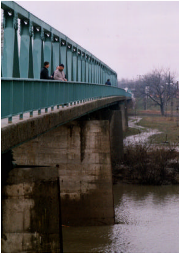
Figure 2 -Sampling from the Bridge at Trivadar, Hungary
